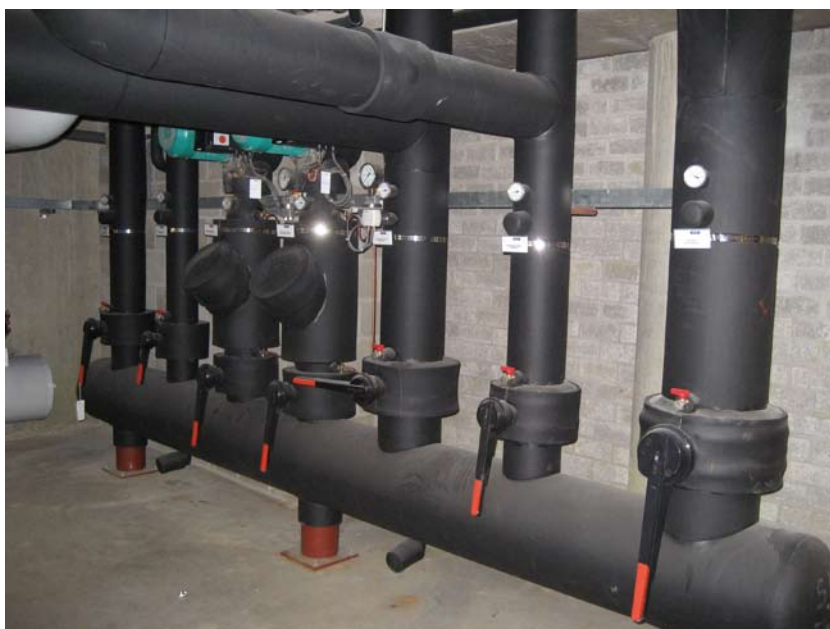
With Armaflex cold installations are reliably protected against energy losses
